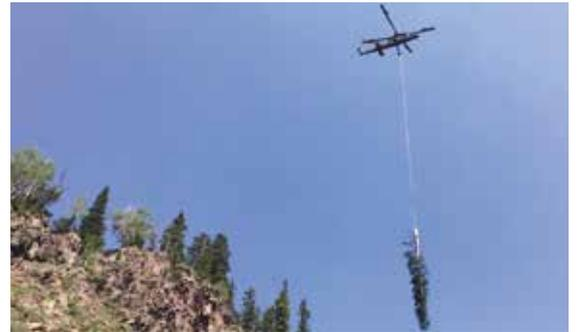
Tree removal by helicopter is the only practical method of vegetation clearing in the high mountain terrain. By law, wherever a helicopter bearing load will cross the highway, the road must be closed.
