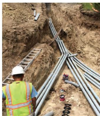
The underground tie line in the Illium Valley (seen here under construction) gives SMPA engineers, operations crews and dispatchers another option to restore power when nature strikes.
