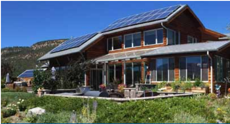
Construction on the 35-acre plot began in 2010 and made use of only local materials as well as local labor and craftsmen.
