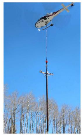
Mountain Blade Runner Chief Pilot, John Whedon lowers a power pole into position using radio guidance from SMPA crews on the ground. In many cases, the pilot cannot see the hole into which the power pole is being seated. Clear communication with ground crews is essential.
