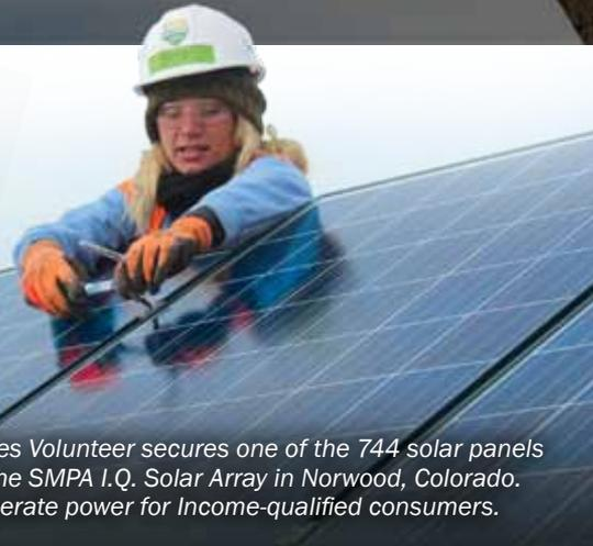
A GRID Alternatives Volunteer secures one of the 744 solar panels which comprise the SMPA I.Q. Solar Array in Norwood, Colorado. The array will generate power for Income-qualified consumers.
