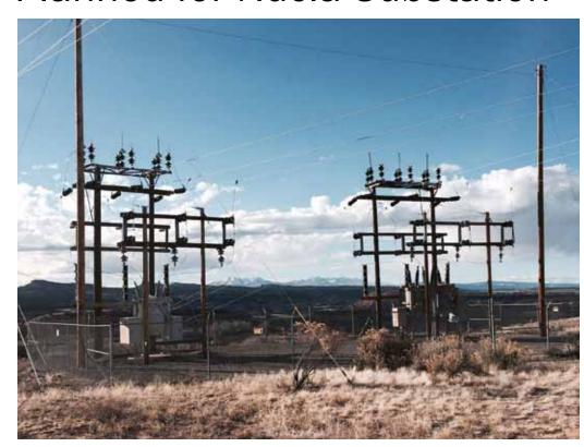
Nucla Substation: Located just southwest of the town of Nucla, the Nucla Substation will soon see major upgrades as SMPA kicks off the West End Reliability project. Improvements include the installation of a new transformer and modern breakers and protective devices. The project will boost power reliability for SMPA members in the region. Photo by Terry Daley, Manager of Engineering
