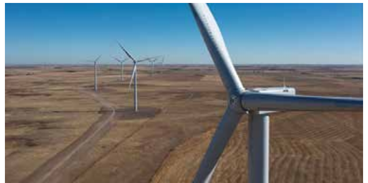
The Niyol Wind Energy Center features 74 wind turbines capable of generating up to 200 megawatts of clean, renewable energy.
