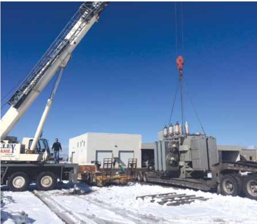
**New Nucla Transformer:** The new transformer bound for the Nucla Substation, along with an identical spare unit, were delivered in mid-February. The original transformer was damaged in a lightning strike in the summer of 2013. The spare unit will serve as a dedicated backup transformer for the West End.
